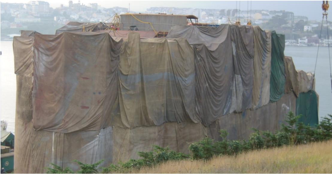
**Hull and Ships sides to be sandblasted and painted prior to launch**
