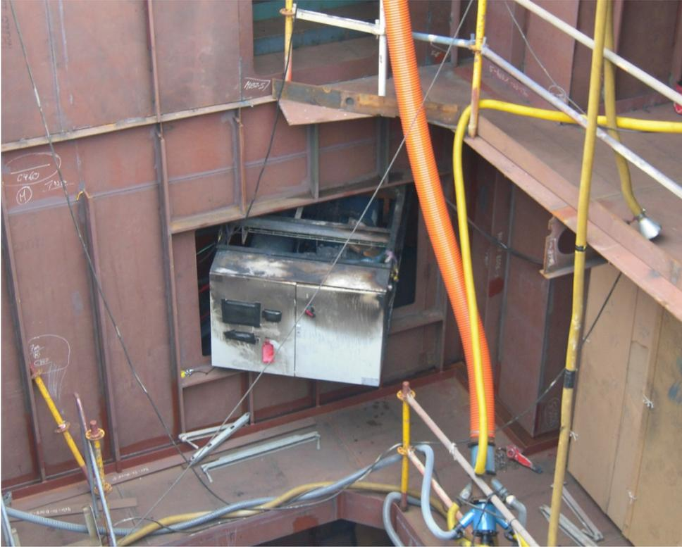
**Replacement of damaged steel bulkhead, due to fire incident**
