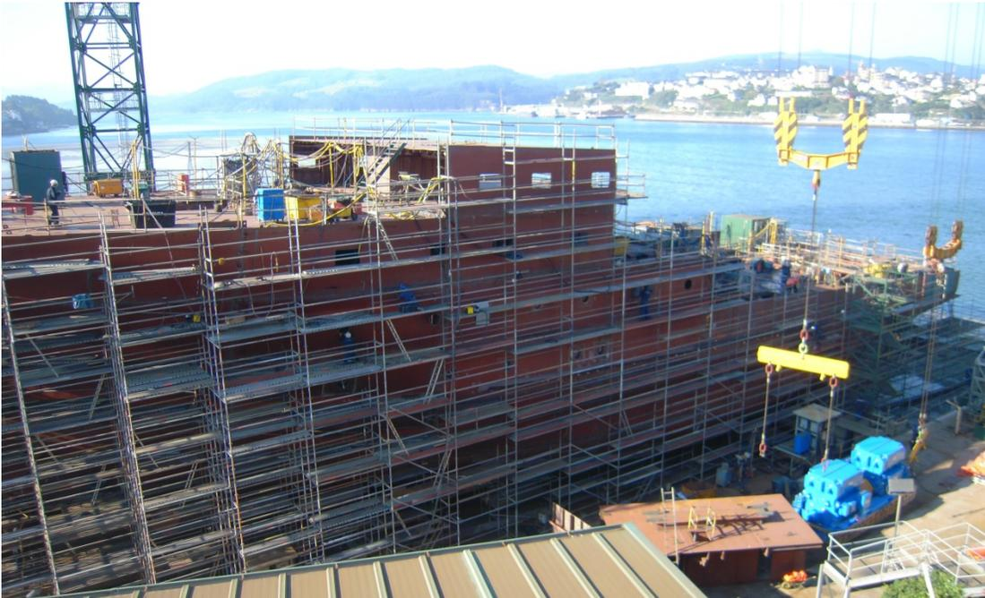
**BL 17 (stern) lower part assembled – full length of vessel now on slipway**
